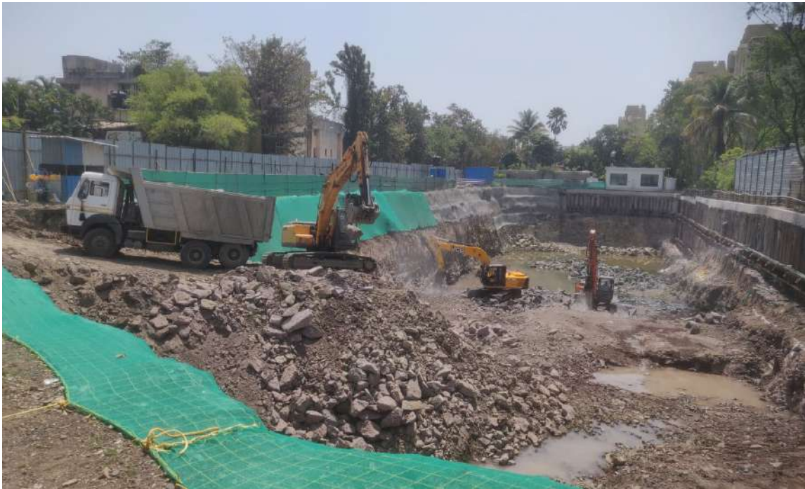
CURRENT SITE STATUS
