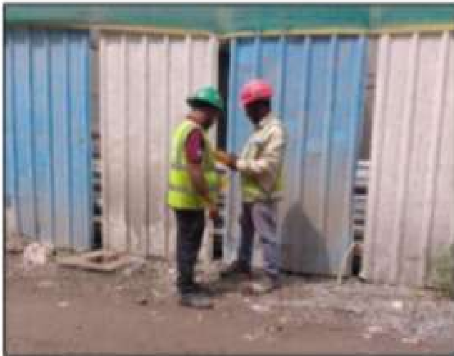
Earthing Inspection Activity
