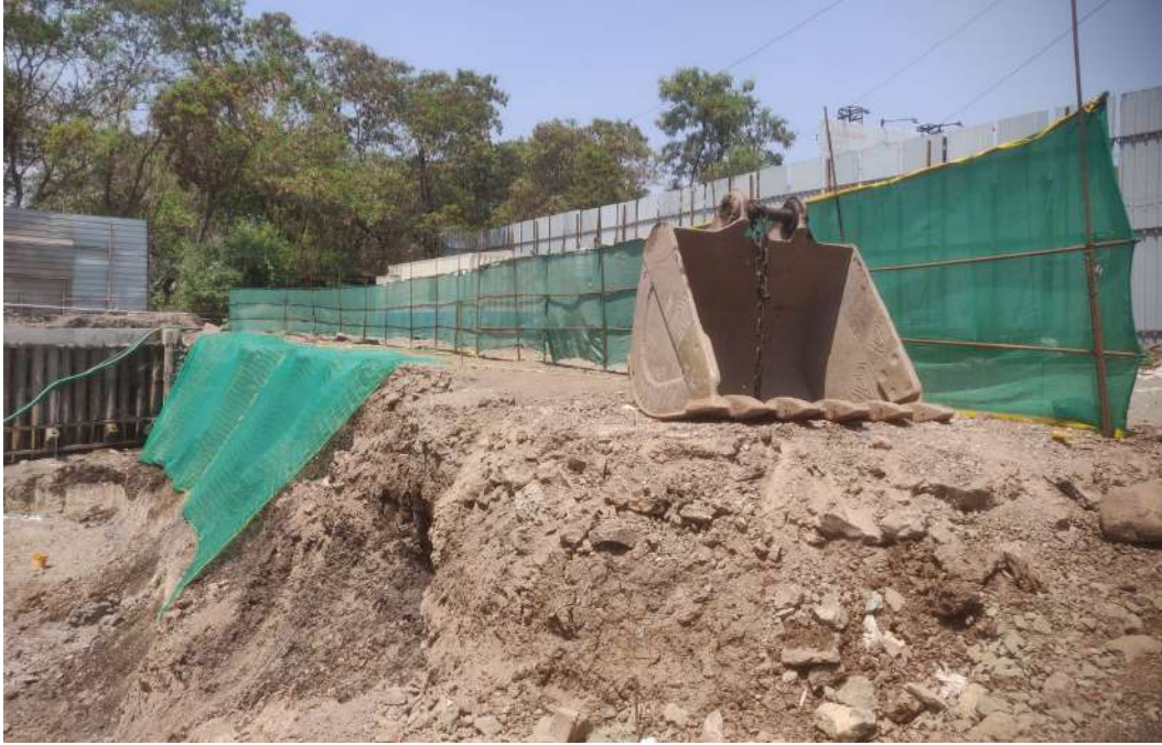
EXCAVATION SIDE PROTECTION
