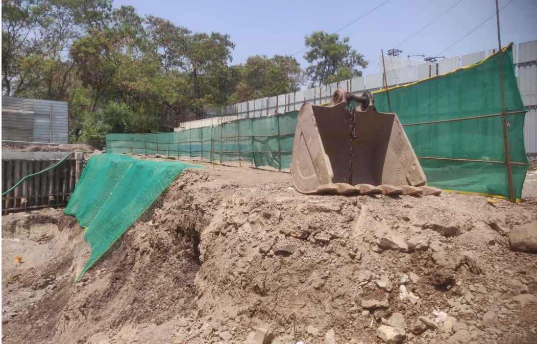
EXCAVATION SIDE PROTECTION
